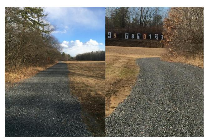
Punctured tires should now be a thing of the past after a few, much needed loads of finer stone were placed on the access road under Mike McGill's direction
